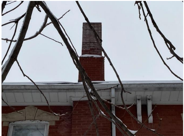
Plate 28: West chimney of west elevation
