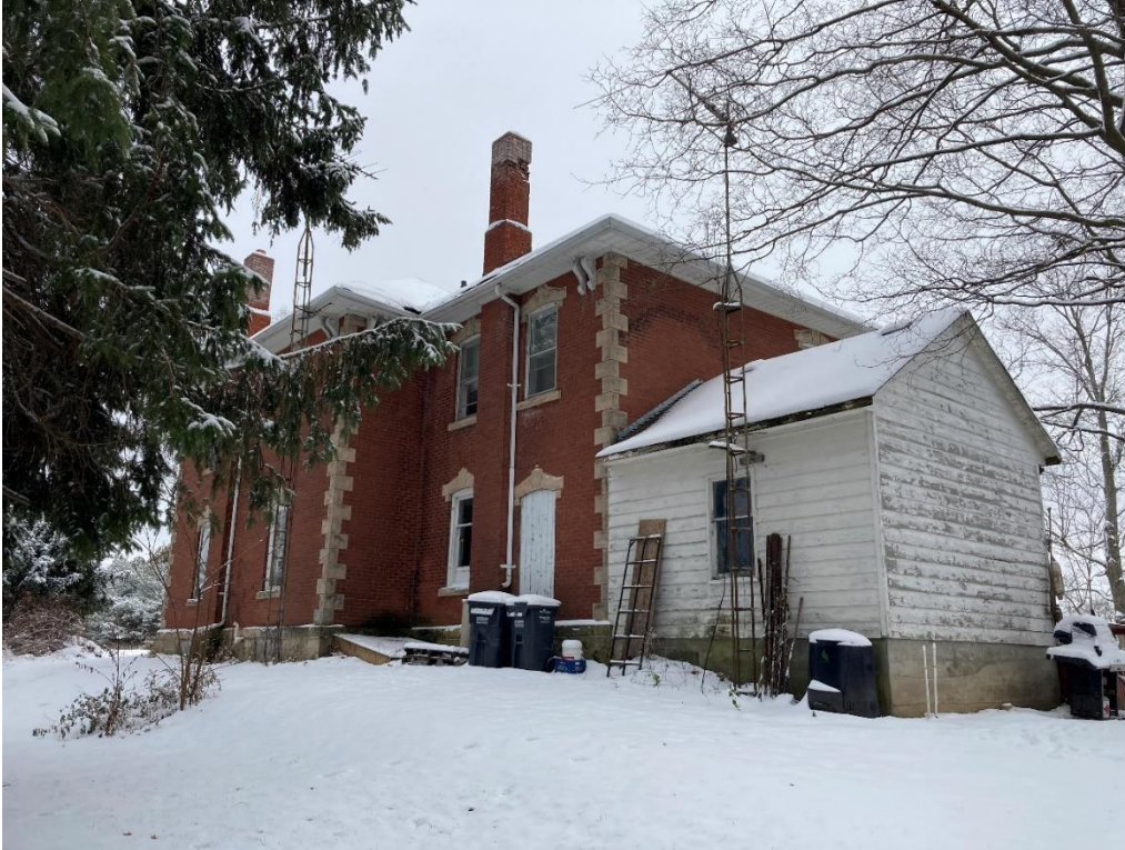
Plate 15: Oblique view of west and south elevations.
