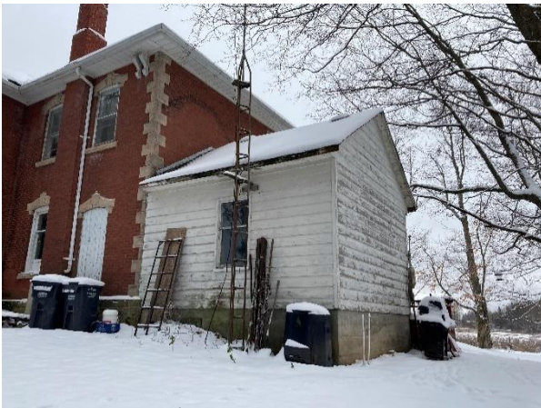
Plate 35: East and south elevations of rear addition
