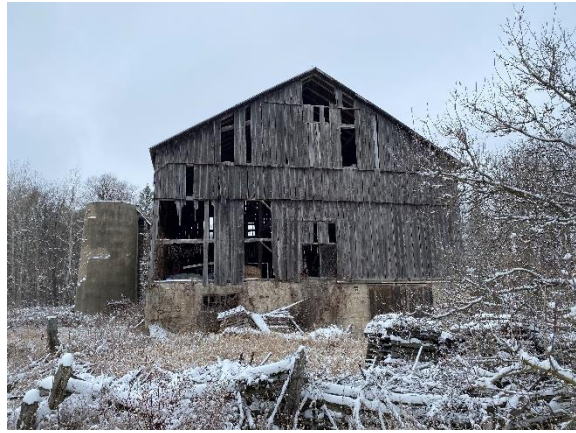
Plate 38: Southeast elevation of the barn
