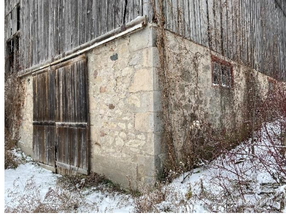
Plate 42: Stone quoins of foundations
