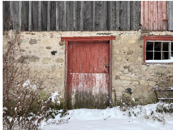
Plate 44: Detail of door and window of barn
