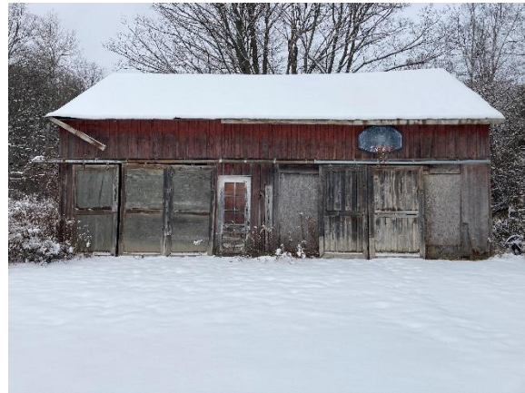
Plate 46: Board-and-batten driven shed
