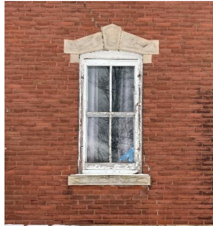
Plate 18: Main block window example
