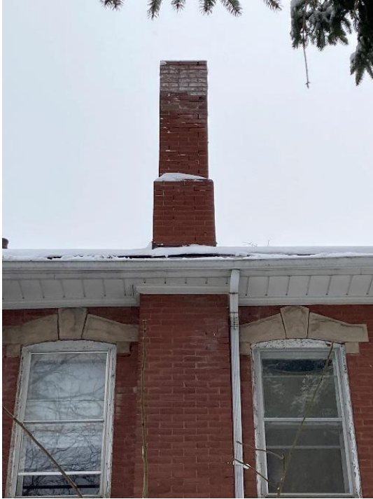
Plate 29: South chimney on west elevation
