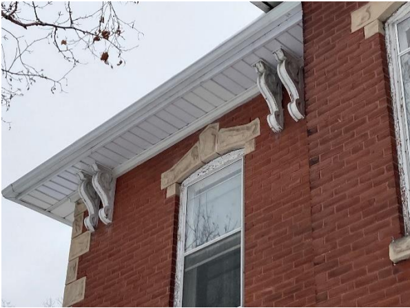
Plate 17: Overhanging eaves and paired bracket detail
