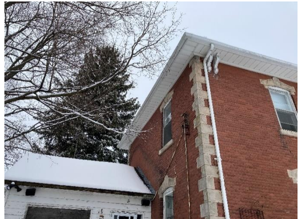
Plate 34: Second floor and eaves of south elevation
