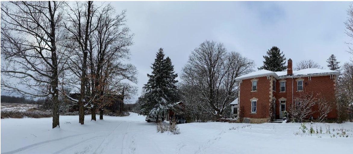
Plate 9: View up the driveway towards house, facing southwest
