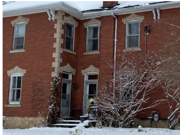
Plate 20: Perpendicular entrance doors on east elevation
