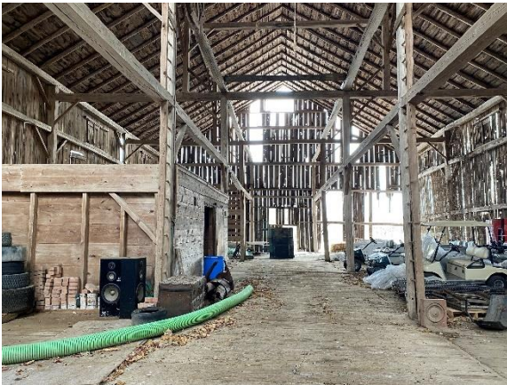
Plate 39: Interior frame structure of the barn
