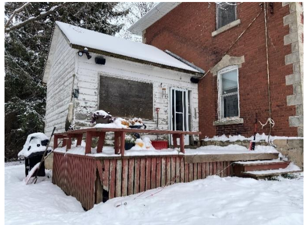
Plate 36: South and west elevations of rear addition
