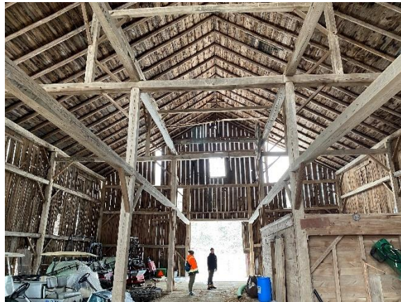
Plate 40: Interior frame structure of the barn
