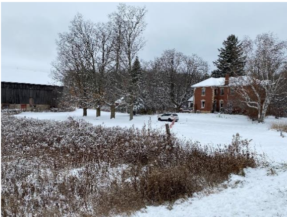
Plate 10: View from Main Street, looking west, across the driveway towards the barn and farmhouse
